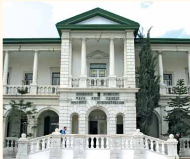
The Lemesos (Limassol) District Administration offices.
