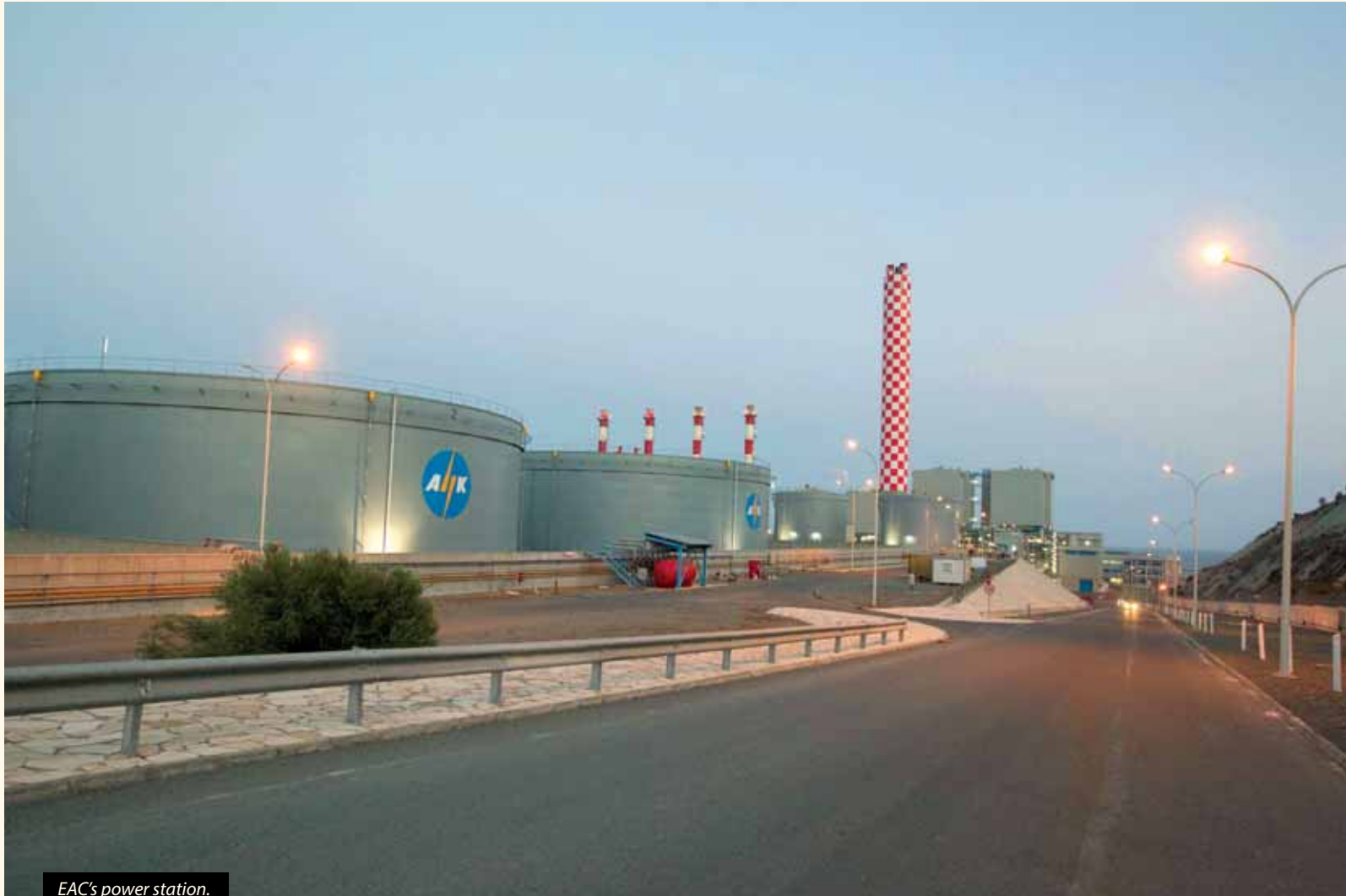
EAC's power station.
