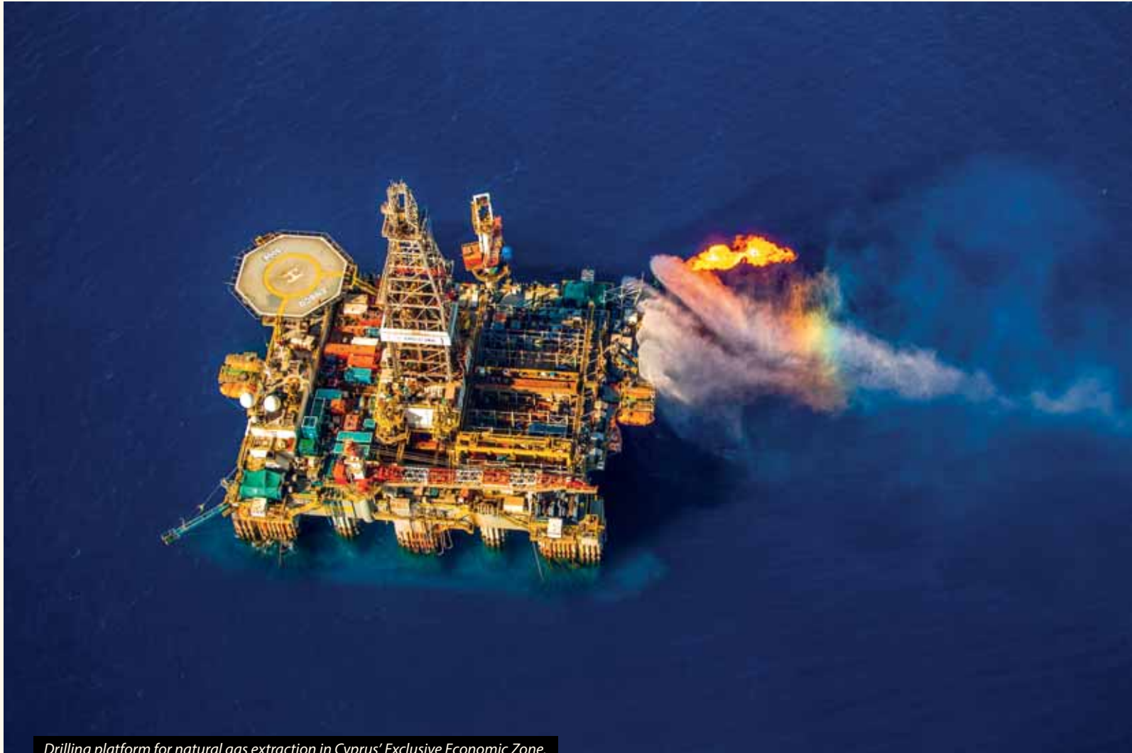
Drilling platform for natural gas extraction in Cyprus' Exclusive Economic Zone.
